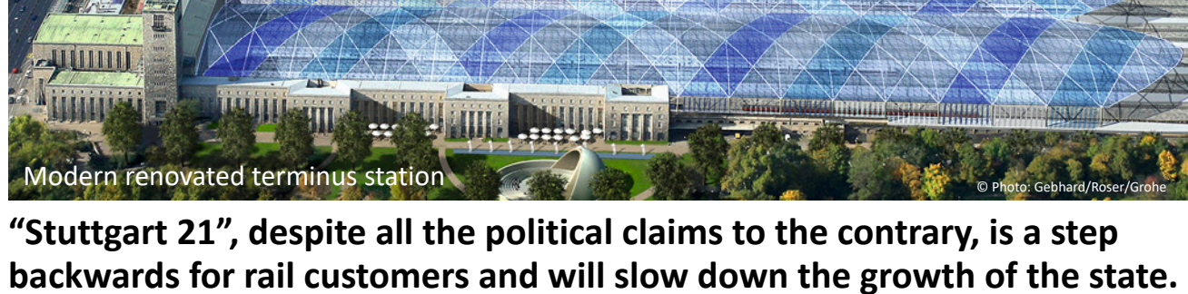
Modern renovated terminus station
